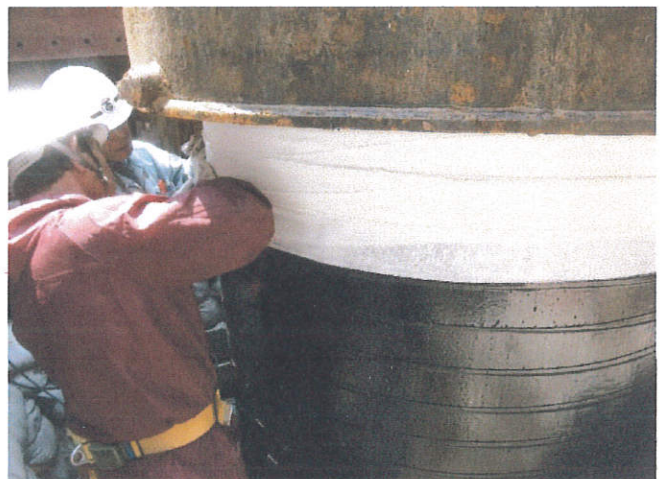
④ Then, wrap Magicawrap with 5 layers for anti-corrosion
