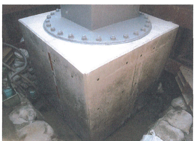
⑥ Finally, make the concrete base.
