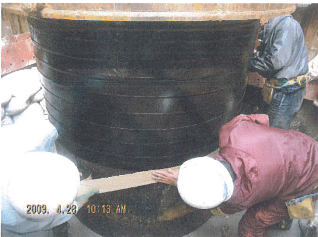
③ Wrap Butyl roll on the whole pipe, pushing it into the unevenness of the surface.
