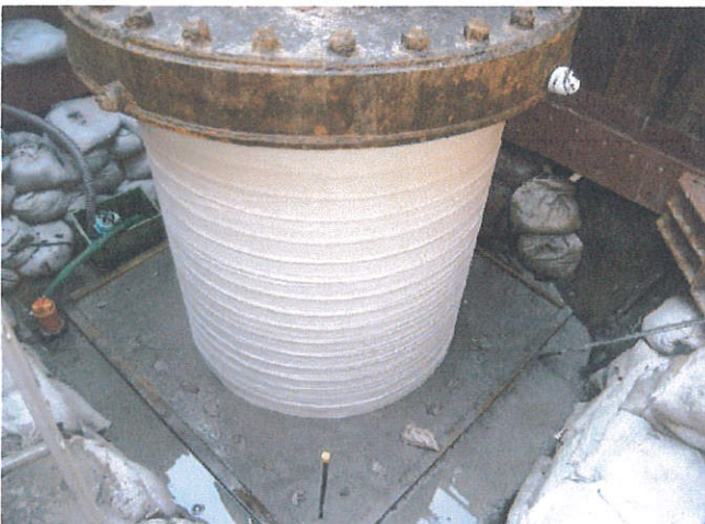
⑤ After wrapping the Magicawrap, squeeze it at the same direction to make the resin even in the Magicawrap.
