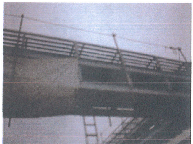
⑩ Have done the same work on the overpass piping
