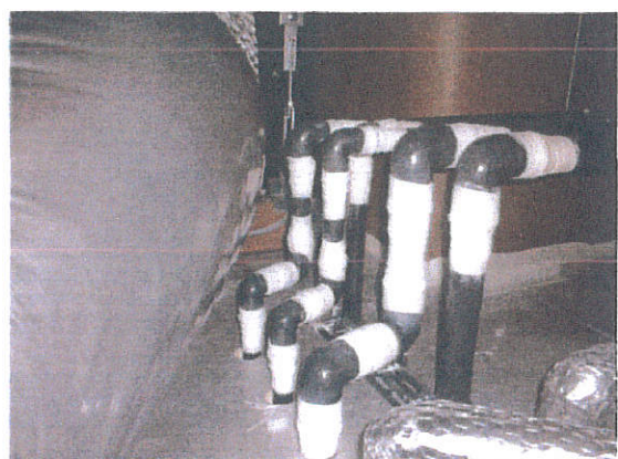
⑥ Have finished the reinforcement on all the joints
