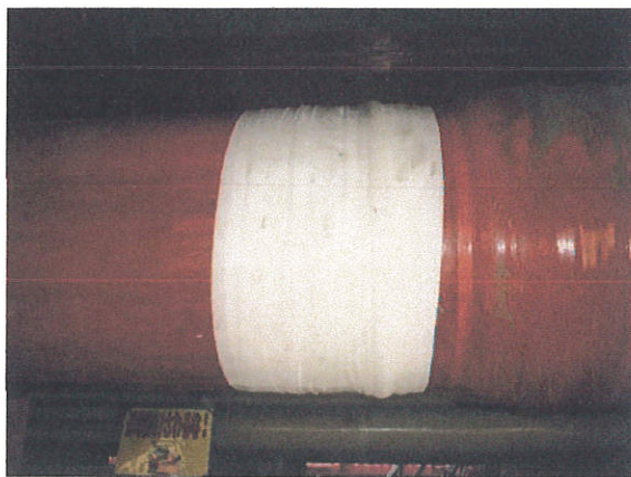
⑧ Then, wrap the Magicawrap and squeeze 1-2 minutes at the same direction.
